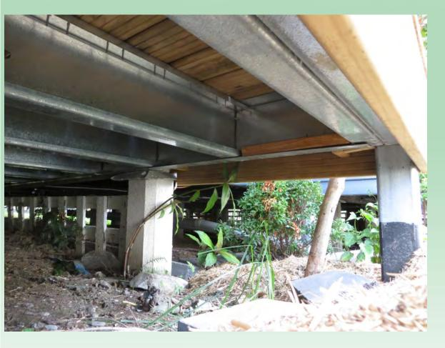
ACQ treated pine decking direct to gal steel joists
