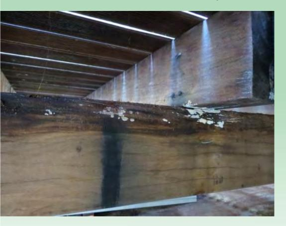
For hardwood, generally Durability Class 1 limits on untreated sapwood (CTIQ, AS 2082) max 1/3<sup>rd</sup> of edge etc.
