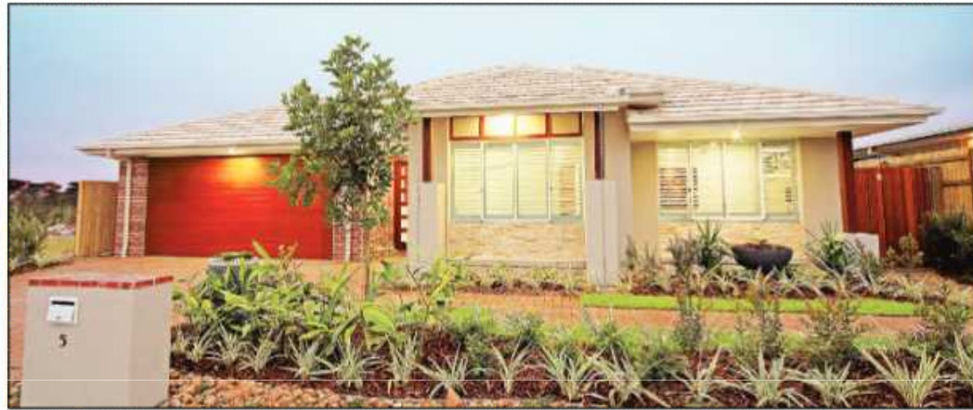
AUSBUILD'S Everton with an Eight Star Energy Efficiency rating is now open as a display home at the Eprapah estate at Victoria Point.
