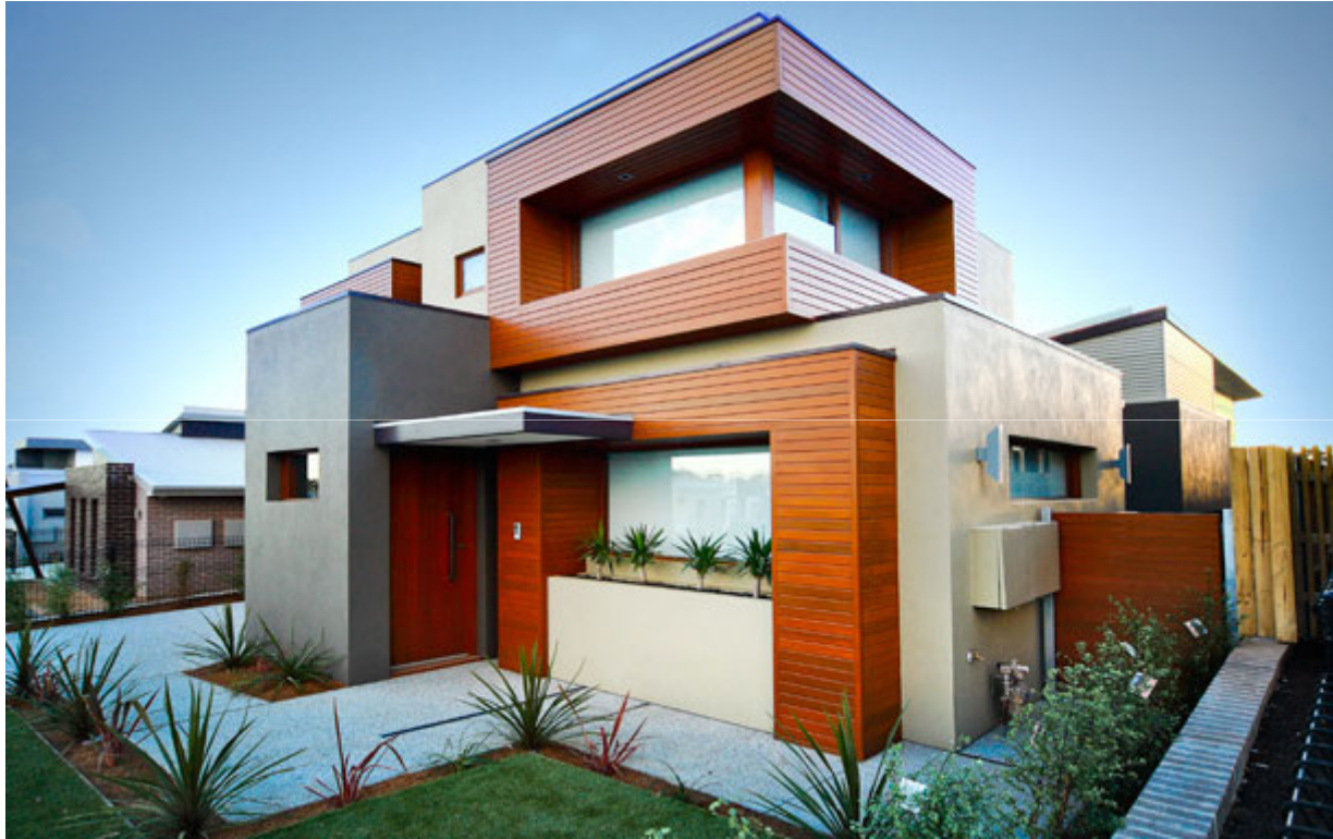
Clay Street Eco Haus
